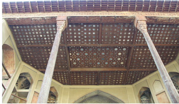
Figure 8: The north porch of Hasht Behesht Palace. The porch length is divided to three parts by the columns, and the proportion between its divisions is golden section.
